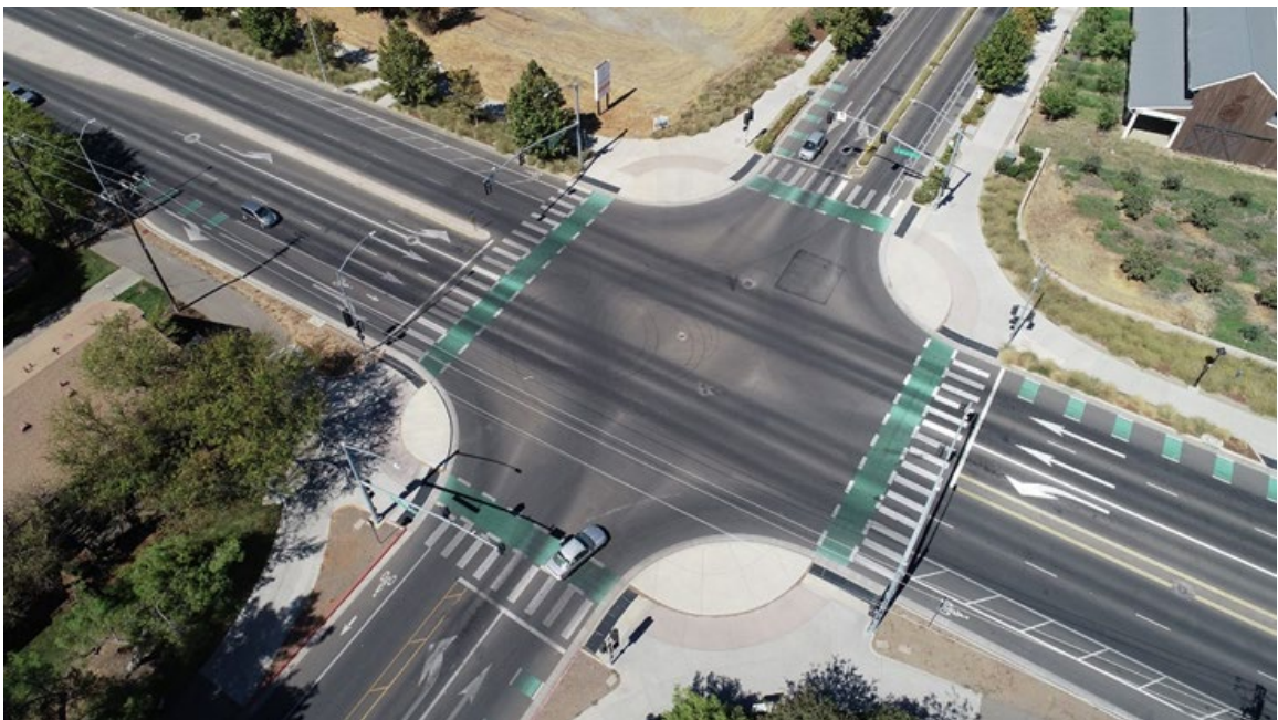
Figure 6: Protected Intersection Example (Davis, California)
