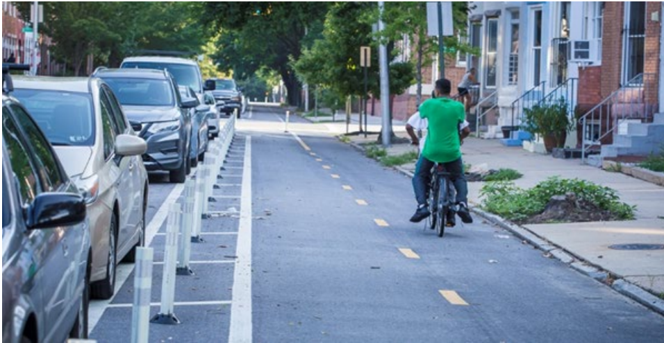
Figure 4. Parking Protected Two-Way Bicycle Lane
